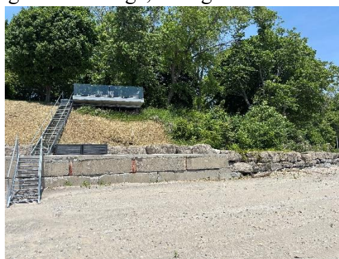
Image 4: Inaccessible rock wall within subject property, along eastern edge, facing north.
