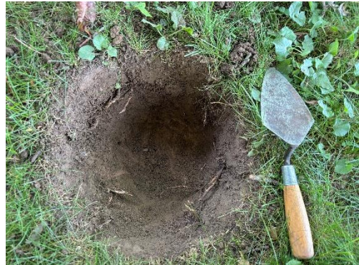
Image 10: Typical test pit.
