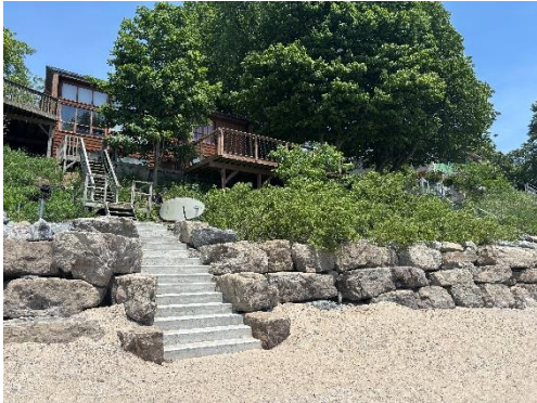
Image 7: Inaccessable rock wall, steeply sloping area and beach within southwestern corner of subject property, facing northeast.
