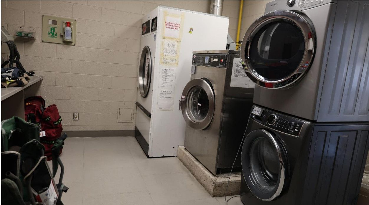
Figure 5 - Gear Washing Room
