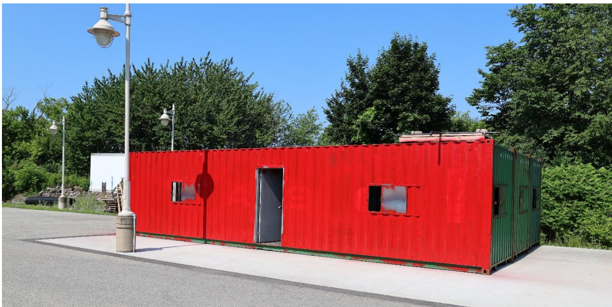
Figure 2: Training Facility - converted sea containers.
