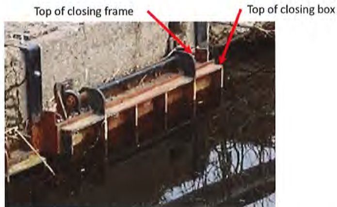
Figure 1 Existing gate after being rehung
