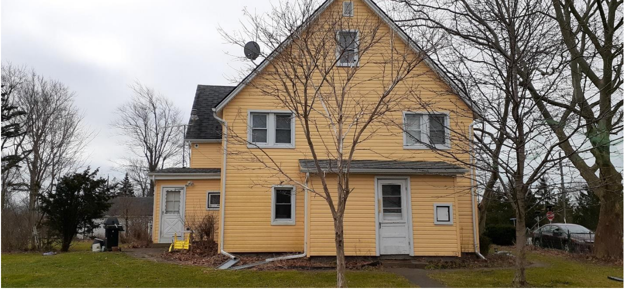
Fig. 15 North side of house, 5446 Sherkston Road
