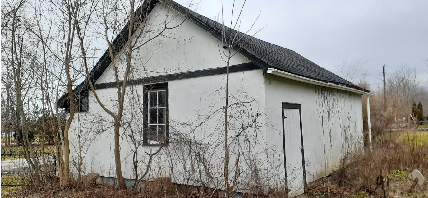
Fig. 3 Old Blacksmith Shop east side 5446 Sherkston Road
