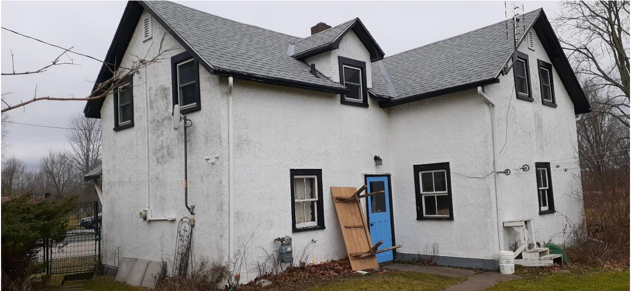
Fig. 7 Old stable south and east sides
