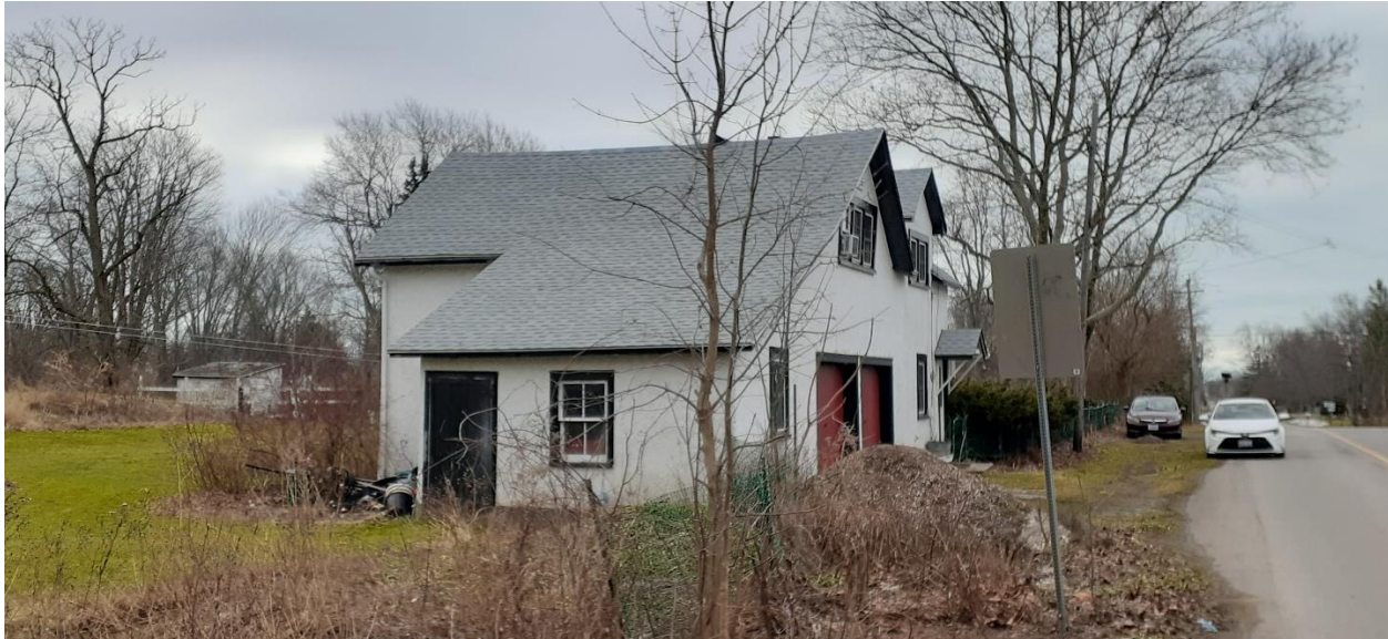
Fig. 9 Old stables north side
