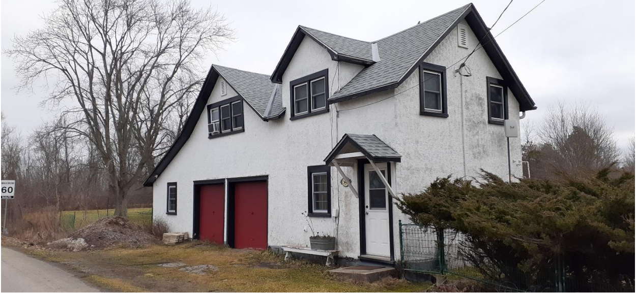
Fig. 6 Old stables west and south sides
