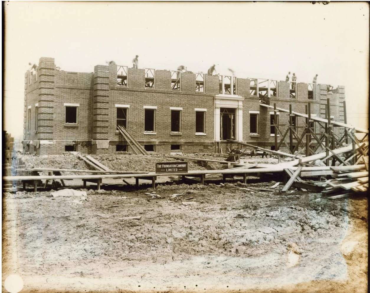
Appendix 1 – Photograph, ca. 1917, from the collection of M. Hili, scanned 2025
