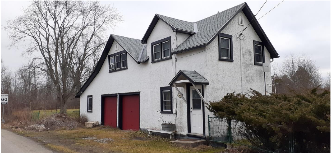
Fig. 6 Old stables west and south sides
