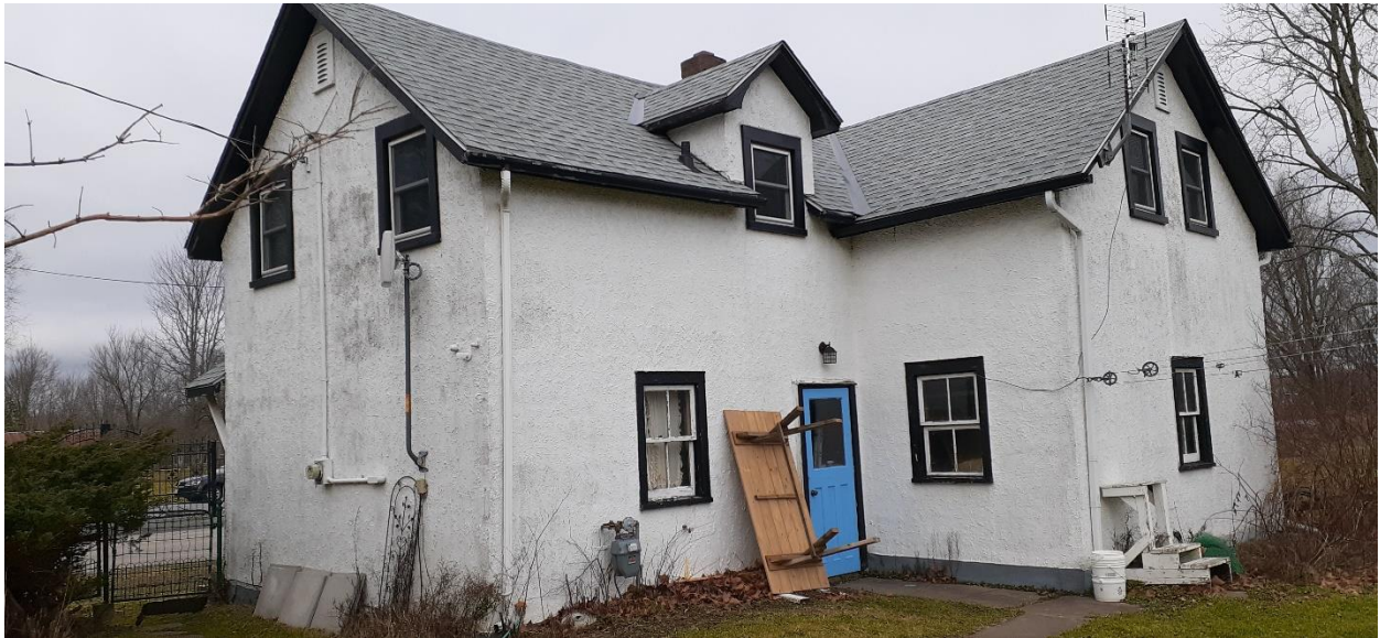
Fig. 7 Old stable south and east sides
