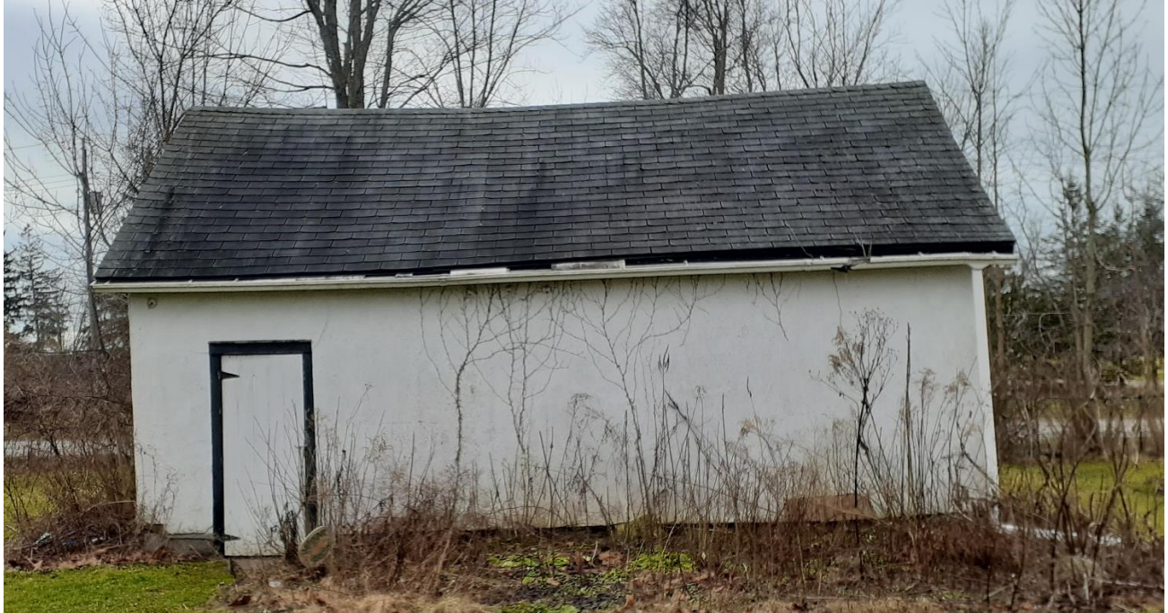
Fig. 4 Old Blacksmith Shop north Side 5446 Sherkston Road
