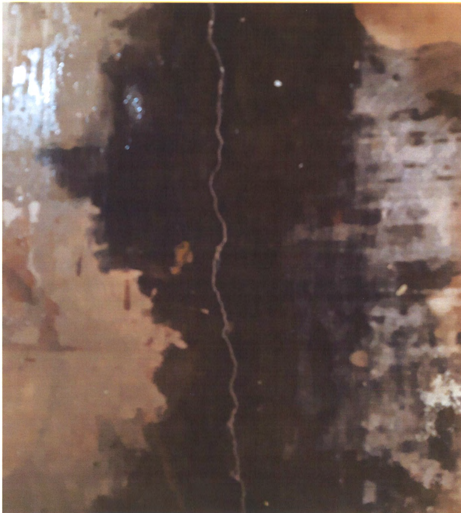
Crack in basement floor
