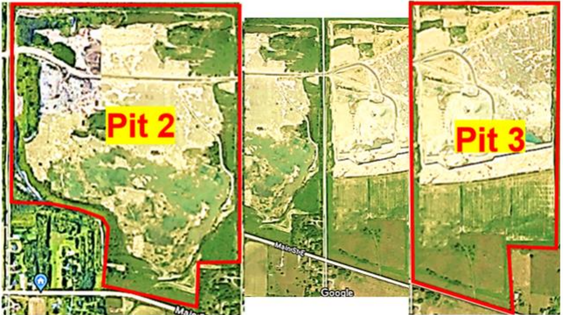
Figure 2 Pit 2 and Pit 3
