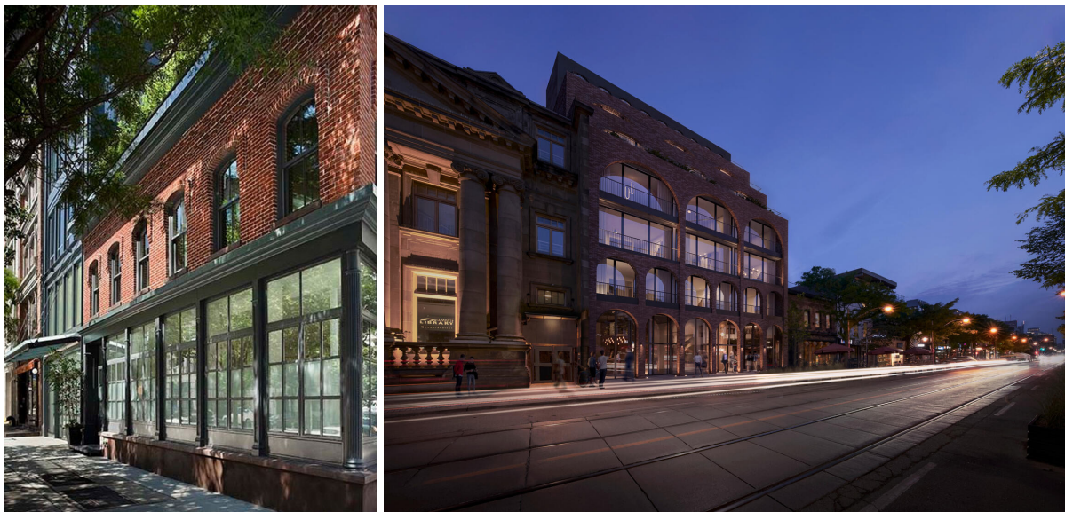
Figure 5 : Examples of façade articulation through the use of upper level step-backs, materials and colours that helps to break-up building massing and provide visual interest. Image credit: (Left) Turett Collaborative Architects - Tribeca Townhouse, New York; (Right) BDP Quadrangle – Biblio, Toronto
