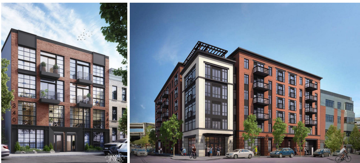
Figure 15 : Building with integrated balconies. Image credits: (Left) Infocus Architects - 340-342 Chauncey Street in Brooklyn; (Right) SERA Architects - NW 19th & Quimby in Portland Oregon
