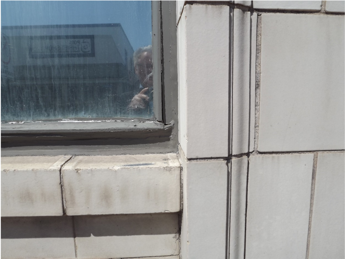
Deteriorated corner of frame
