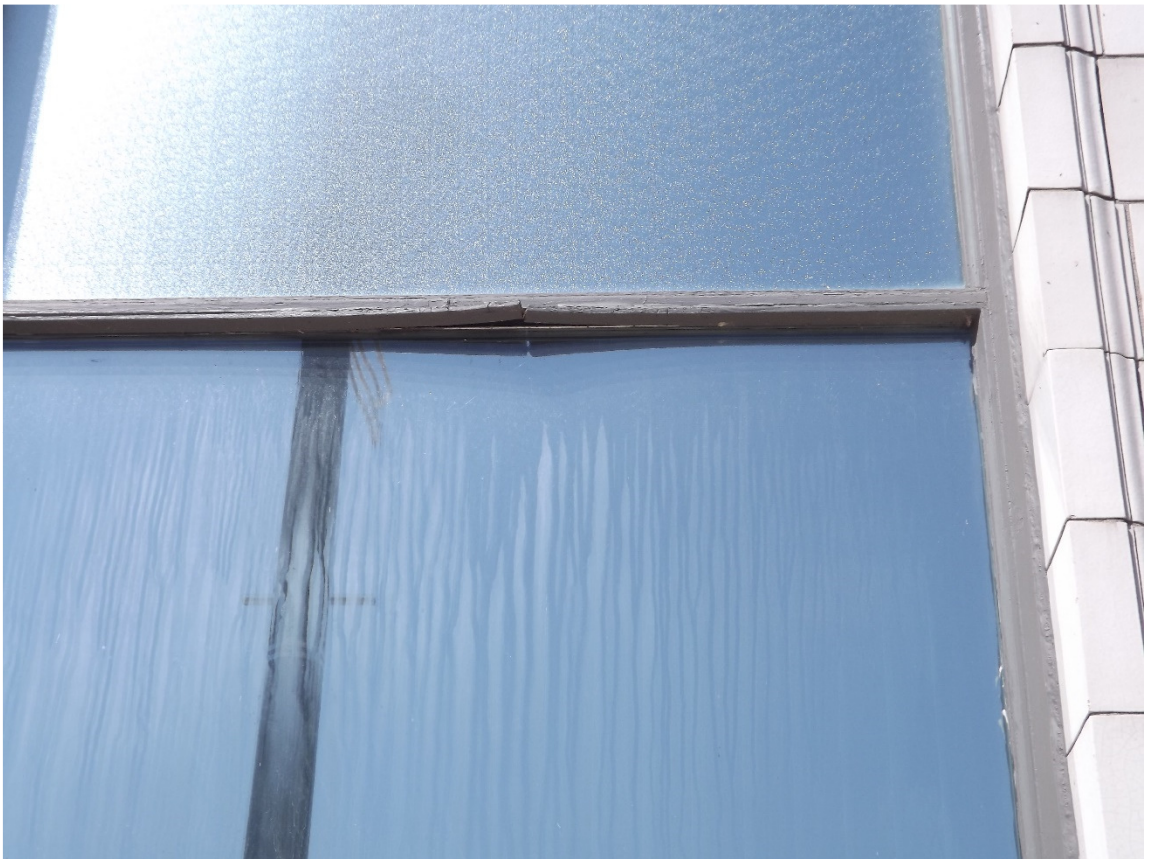
Failing horizontal mullion
