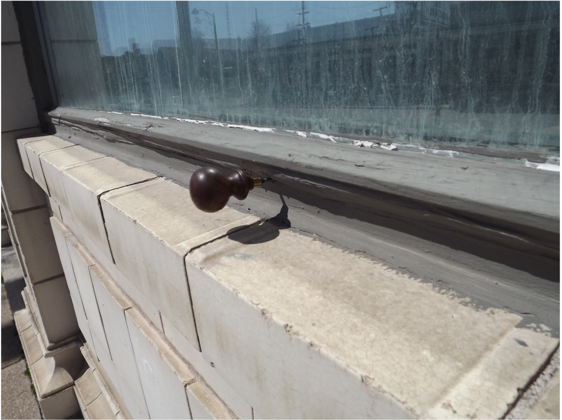
Awl with 5" blade inserted into window sill, south facade
